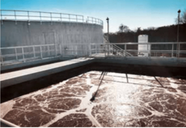
Digester System SOURCE: ADI SYSTEMS
